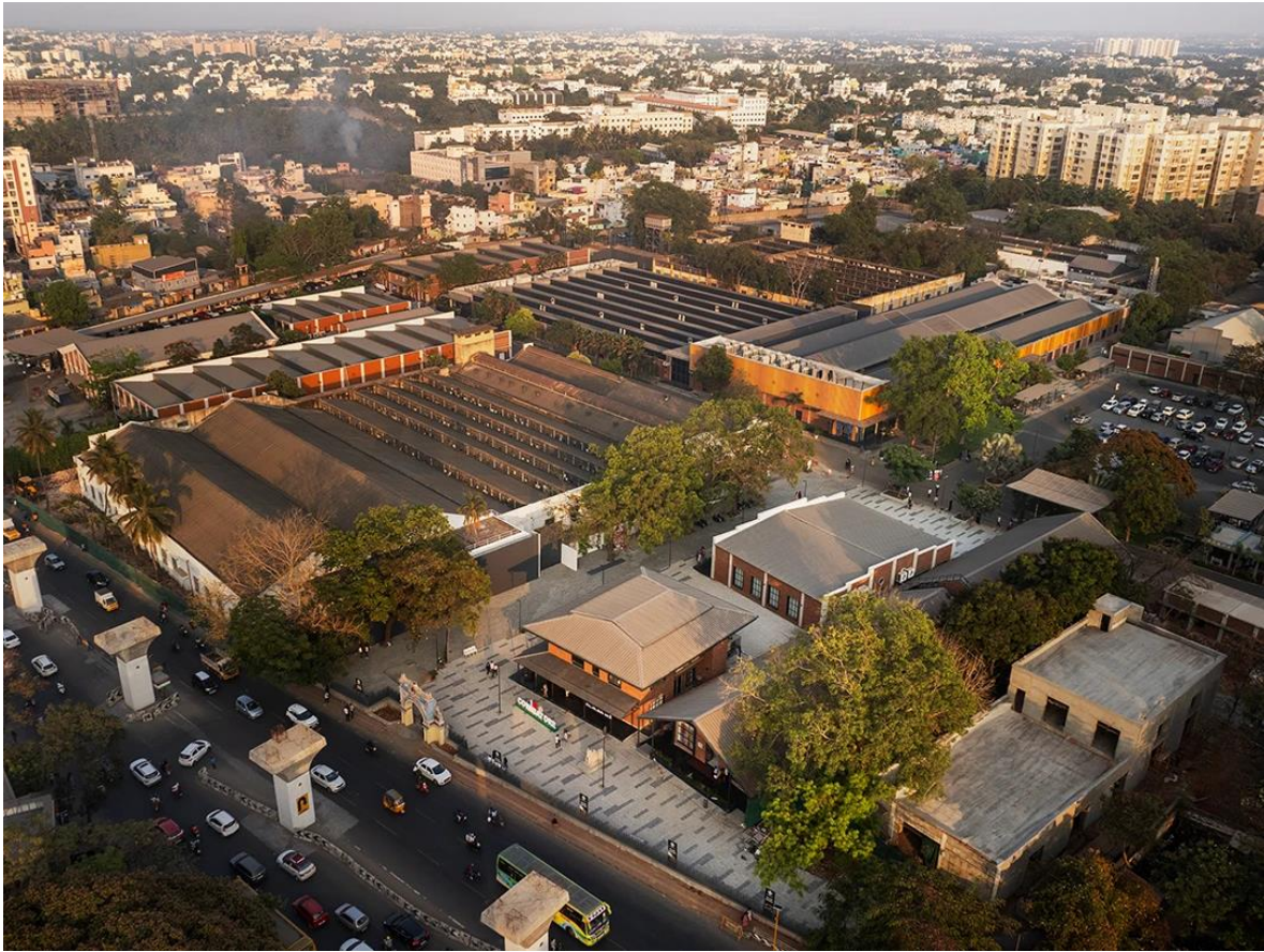
Figure 8 Aerial view of Lakshmi mills rejuvena-tion_© https://www.studiolotus.in/projects/lakshmi-mills-redevelopment
